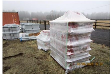
AID MCPH2 - Stored Material; gate valves + meter boxes 01-06-25
