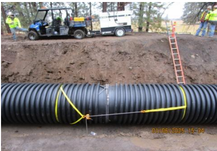
AID MCPH2 - Sta. 866+93 54-IN pipe, field joint electrofusion in process 01-06-25
