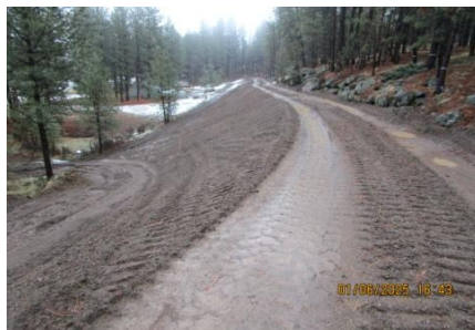
AID MCPH2 - Sta 817+50 embankment fill complete 1.5-IN minus 01-06-25
