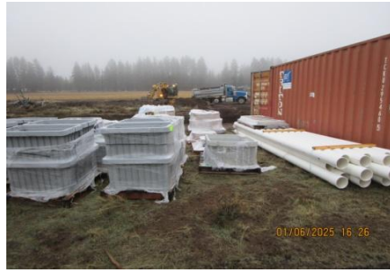
AID MCPH2 - Stored Material; meter boxes + valve riser pipe 01-06-25
