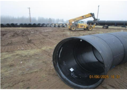
AID MCPH2 - Stored Material 54-IN RSC400 profile wall pipe and fittings (2) 01-06-25
