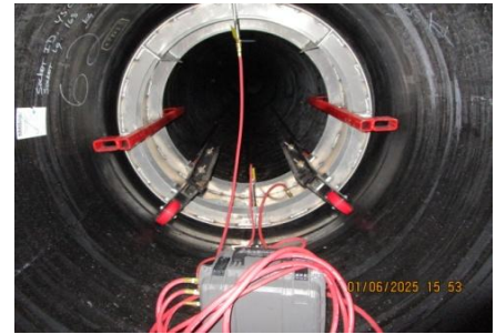
AID MCPH2 - 54-IN pipe, air test equipment 01-06-25
