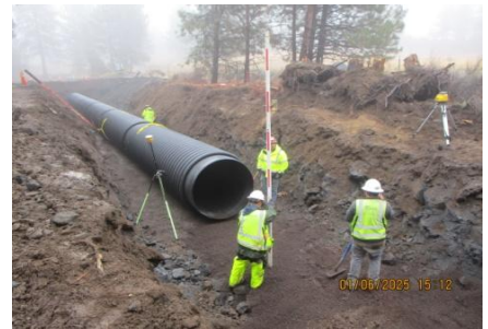
AID MCPH2 - Sta. 866+55 54-IN pipe, pipe setting + grade check in process 01-06-25
