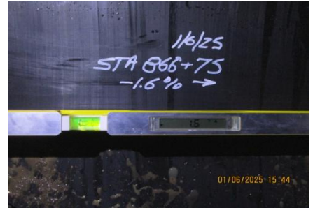
AID MCPH2 - Sta. 866+75 54-IN pipe, QA pipe slope measure 01-06-25
