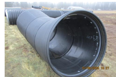
AID MCPH2 - Stored Mtrl 54-IN RSC400 profile wall pipe and fittings (1) 01-06-25
