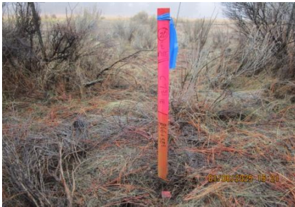
AID MCPH2 - Sta. 866+58 54-IN pipe construction staking, cut to invert 7.51-FT 01-06-25
