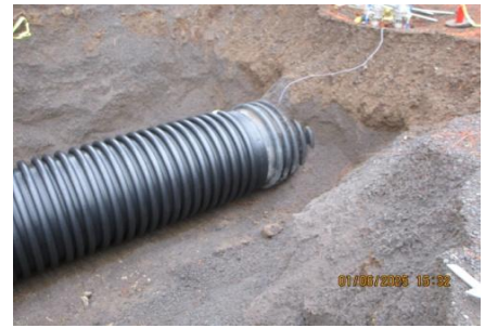
AID MCPH2 - Sta. 867+97 54-IN pipe, POC point-of-connection ex. 54-IN pipe 01-06-25
