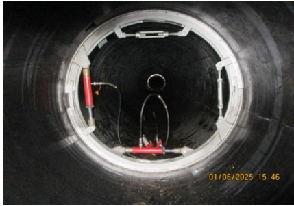
AID MCPH2 - 54-IN pipe, internal joint expander 01-06-25
