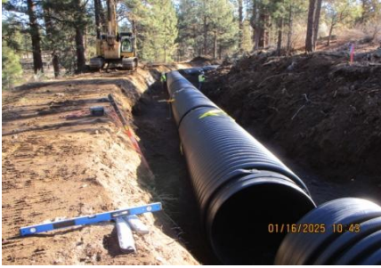
AID MCPH2 - Sta 854+00 54-IN profile wall HDPE pipe installed 01-16-25
