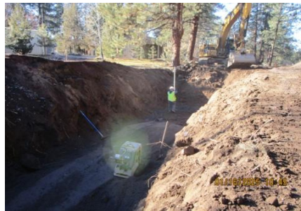
AID MCPH2 - Sta 852+75 54-IN profile wall HDPE pipe trench excavation 01-16-25
