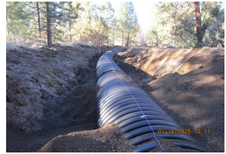
AID MCPH2 - Sta 859+50 54-IN profile wall HDPE pipe installed 01-16-25
