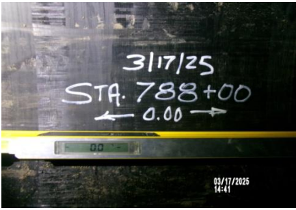
AID MCPH2 - Sta 788+00 54-IN ID profile wall HDPE pipe QA pipe slope measurement 0.0% level 03-17-25
