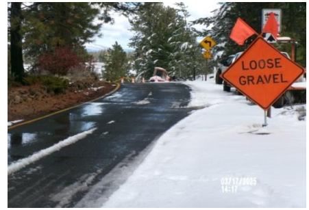
AID MCPH2 - Sta 791+00 right Woodside Road temp gravel surface access 03-12-25
