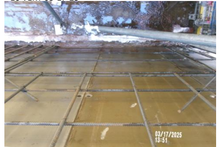
AID MCPH2 - Sta 718+00 Intake Structure wall reinforcing steel, weir wall at blockout, #5 @ 18 HOR + #5 @ 16 VERT + (1) add ea side + top 03-17-25
