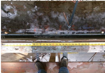
AID MCPH2 - Sta 718+00 Intake Structure wall reinforcing steel, weir wall typ, #5 @ 16 VERT 03-17-25
