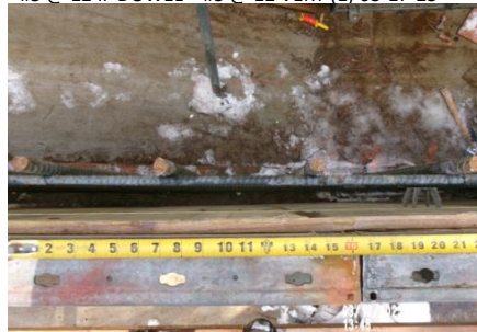
AID MCPH2 - Sta 718+00 Intake Structure wall reinforcing steel, weir wall slope, #7 @ 8 VERT 03-17-25
