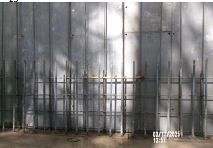
AID MCPH2 - Sta 718+00 Intake Structure wall reinforcing steel, outside wall, #8 @ 7 OF DOWEL + #5 @ 12 IF DOWEL + #5 @ 12 VERT (1) 03-17-25
