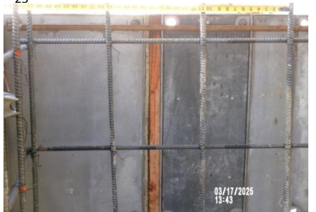
AID MCPH2 - Sta 718+00 Intake Structure wall reinforcing steel, weir wall, #5 @ 18 HOR + #5 @ 16 VERT 03-17-25
