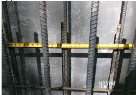
AID MCPH2 - Sta 718+00 Intake Structure wall reinforcing steel, outside wall, #8 @ 7 OF DOWEL + #5 @ 12 IF DOWEL + #5 @ 12 VERT (2) 03-17-25
