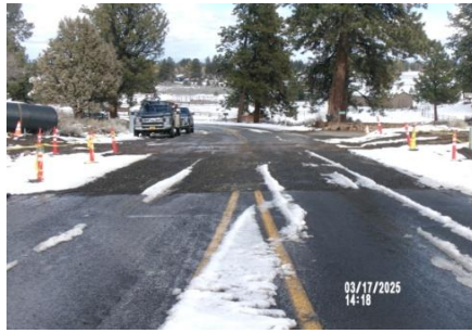
AID MCPH2 - Sta 791+00 Woodside Road Type B Trench backfill + temp gravel surface access 03-12-25
