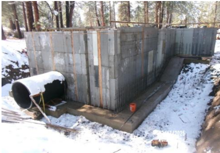
AID MCPH2 - Sta 718+00 Intake Structure wall form and wall reinforcing steel in process (1) 03-17-25
