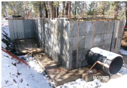
AID MCPH2 - Sta 718+00 Intake Structure wall form and wall reinforcing steel in process (2) 03-17-25
