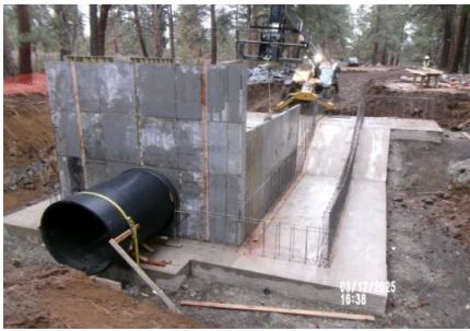
AID MCPH2 - Sta 718+00 Intake Structure wall form erection 03-05-25
