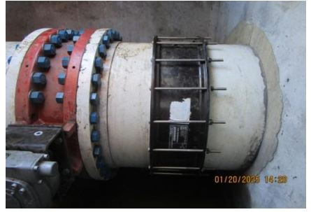
AID MCPH1 - Sta. 1067+09 Warranty Issue 01 36-IN coupler install (6) 01-20-25
