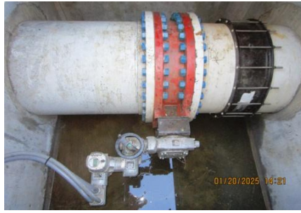
AID MCPH1 - Sta. 1067+09 Warranty Issue 01 36-IN coupler install (7) 01-20-25
