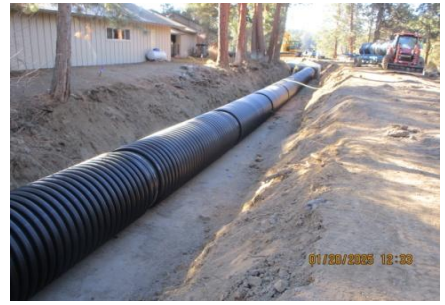
AID MCPH2 Seg2 - Sta. 851+50 54-IN ID profile wall HDPE pipe installed 01-20-25
