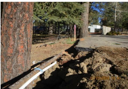
AID MCPH2 Seg2 - Sta. 847+50 existing private water and communication utilities, protect-in-place 01-20-25
