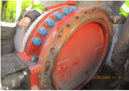
AID MCPH1 - Sta. 1067+09 Warranty Issue 01 36-IN coupler install (4) 01-20-25
