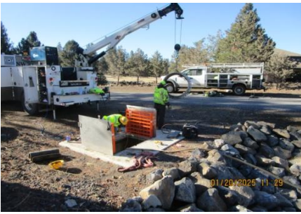
AID MCPH1 - Sta. 1067+09 Warranty Issue 01 36-IN coupler install (1) 01-20-25
