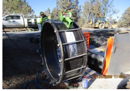
AID MCPH1 - Sta. 1067+09 Warranty Issue 01 36-IN coupler install (5) 01-20-25
