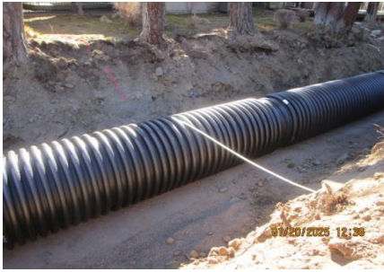
AID MCPH2 Seg2 - Sta. 850+80 existing private water 1-1.4-IN Pex, protect-in-place 01-20-25
