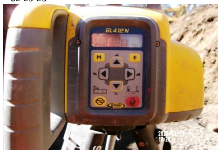
AID MCPH2 - Sta 803+75 54-IN ID profile wall HDPE pipe bed grading 02-25-25
