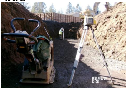
AID MCPH2 - Sta 803+50 54-IN ID profile wall HDPE pipe bedding 02-25-25
