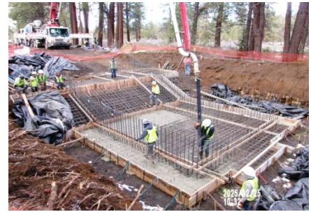
AID MCPH2 - Sta 718+00 Intake Struct Fnd concrete placement, 70 yd3, 50SL428A, 4.500 PSI 02-25-25
