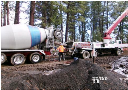
AID MCPH2 - Sta 718+00 Intake Struct Fnd concrete placement, 70 yd3, 50SL428A, boom pump delivery 02-25-25
