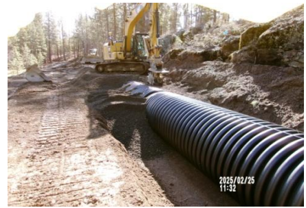
AID MCPH2 - Sta 818+50 54-IN ID profile wall HDPE pipe, initial backfill densification 02-25-25
