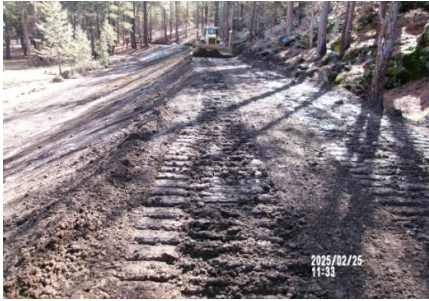
AID MCPH2 - Sta 820+00 54-IN ID profile wall HDPE pipe, final trench backfill, rough grade 02-25-25
