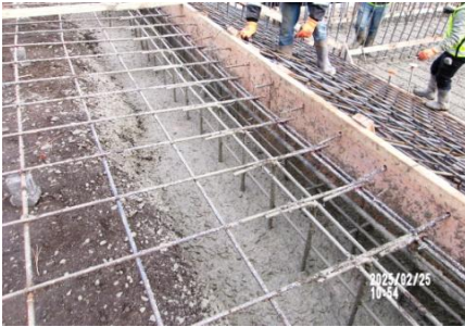
AID MCPH2 - Sta 718+00 Intake Struct Fnd concrete placement, cut-off trench downstream end of approach slab (2) 02-25-25
