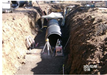
AID MCPH2 - Sta 803+75 54-IN ID profile wall HDPE pipe install and field joint fusion (1) 02-25-25
