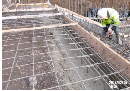
AID MCPH2 - Sta 718+00 Intake Struct Fnd concrete placement, cut-off trench downstream end of approach slab (1) 02-25-25
