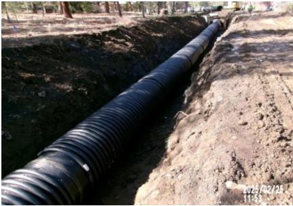
AID MCPH2 - Sta 806+60 54-IN ID profile wall HDPE pipe installed 02-25-25
