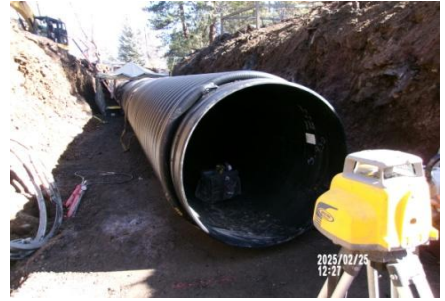
AID MCPH2 - Sta 803+75 54-IN ID profile wall HDPE pipe install and field joint fusion (2) 02-25-25
