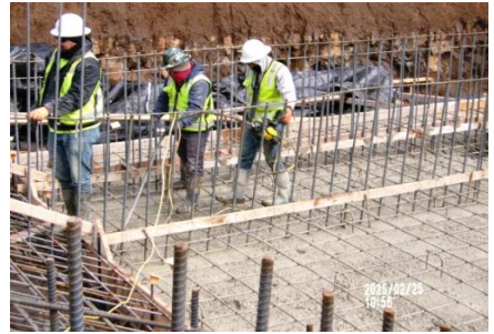
AID MCPH2 - Sta 718+00 Intake Struct Fnd concrete placement, 70 yd3, 50SL428A, high cycle consolidation 02-25-25
