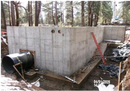
AID MCPH2 Seg2 - Sta. 718+00 Intake Structure wall form removal (1) 04-01-25
