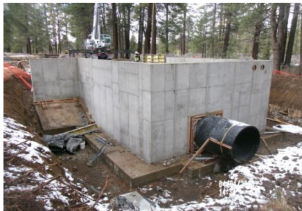
AID MCPH2 Seg2 - Sta. 718+00 Intake Structure wall form removal (2) 04-01-25
