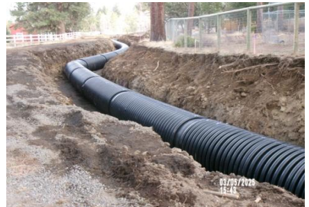
AID MCPH2 - Sta 795+00 54-IN ID profile wall HDPE pipe installed 03-05-25
