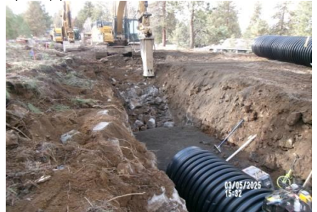
AID MCPH2 - Sta 793+10 54-IN ID profile wall HDPE pipe trench excavation 03-05-25
