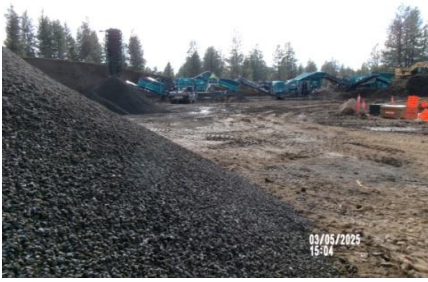
AID MCPH2 - Sta. 720+00 Temp Mtrl Processing Area, 0.75 aggregate processing 03-05-25
