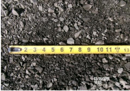
AID MCPH2 - Sta. 720+00 Temp Mtrl Processing Area, stored mtrl, 0.75 SS aggregate Type B Trench backfill mtrl (2) 03-05-25
