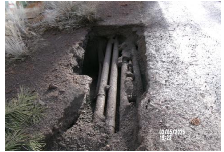
AID MCPH2 - Sta. 791+00 Woodside Rd pothole existing utilities east road shoulder, protect-in-place (1) 03-05-25
