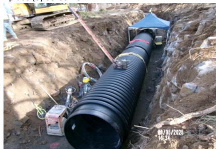
AID MCPH2 - Sta 793+35 54-IN ID profile wall HDPE pipe install and field joint fusion 03-05-25
