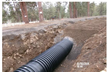
AID MCPH2 - Sta 808+80 54-IN ID profile wall HDPE pipe, initial backfill densification 03-05-25
