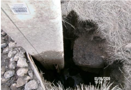
AID MCPH2 - Sta. 791+00 Woodside Rd pothole existing utilities east road shoulder, protect-in-place (3) 03-05-25
