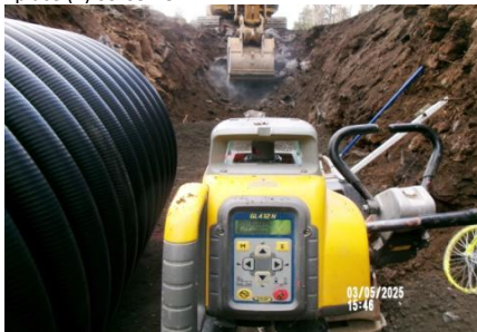
AID MCPH2 - Sta 793+20 54-IN ID profile wall HDPE pipe bed grading 03-05-25
