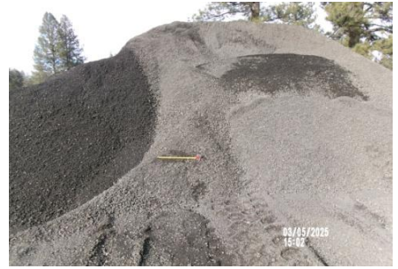
AID MCPH2 - Sta. 720+00 Temp Mtrl Processing Area, stored mtrl, 0.75 SS aggregate Type B trench backfill mtrl (1) 03-05-25
