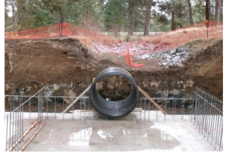
AID MCPH2 - Sta 718+00 Intake Struct Fnd 60-IN ID wall spool template placed (2) 03-05-25
