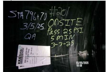
AID MCPH2 - Sta 796+70 54-IN ID profile wall HDPE pipe field joint #201 air pressure test PASS 03-05-25
