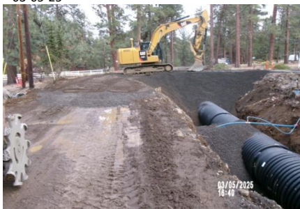
AID MCPH2 - Sta 807+20 54-IN ID profile wall HDPE pipe, Type B trench backfill at access way crossing 03-05-25
