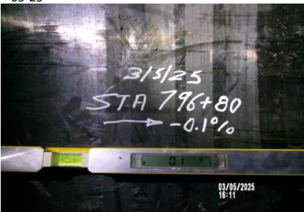
AID MCPH2 - Sta 796+80 54-IN ID profile wall HDPE pipe QA pipe slope measurement -0.1% slope 03-05-25
