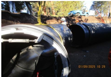
AID MCPH2 - Sta 863+25 54-IN ID 29 degree fabricated fitting install 01-09-25
