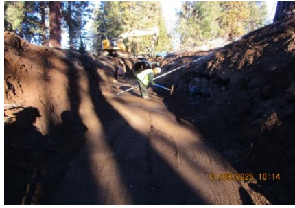
AID MCPH2 - Sta 862+00 54-IN profile wall pipe 0.75-IN aggregate base bedding 01-09-25
