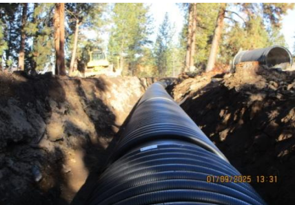
AID MCPH2 - Sta 864+00 54-IN profile wall HDPE pipe installed 01-09-25
