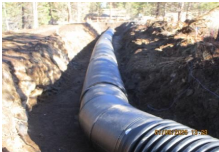
AID MCPH2 - Sta 866+28 54-IN 34 degree bend + profile wall HDPE pipe installed 01-09-25
