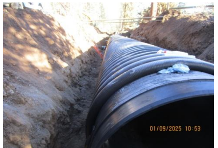
AID MCPH2 - Sta 863+30 54-IN profile wall HDPE pipe setting and electro-fusion 01-09-25
