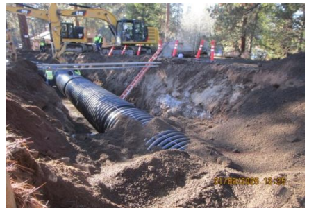
AID MCPH2 - Sta 863+75 54-IN profile wall HDPE pipe setting and electro-fusion 01-09-25
