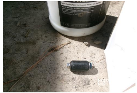
AID MCPH2 Seg2 - Sta. 718+00 Intake Structure, walls, tie hole expansion plugs 04-01-25
