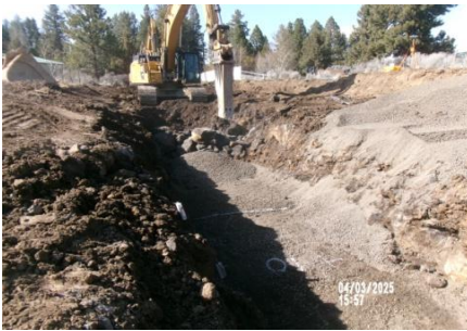
AID MCPH2 - Sta 763+75 54-IN ID profile wall HDPE pipe trench excavation 03-25-25
