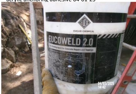
AID MCPH2 Seg2 - Sta. 718+00 Intake Structure, wall collar, approved bonding agent 04-01-25
