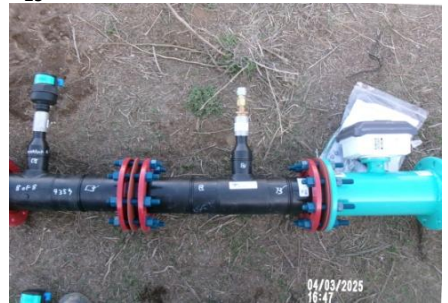
AID MCPH2 - Preassembled 4-In irrigation turnout assembly flow meter + Air Chuck + ARV 04-03-25
