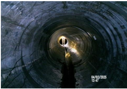
AID MCPH2 - Sta 790+85 54-IN ID profile wall HDPE pipe QA ovality measurements after backfill 04-02-25
