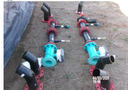
AID MCPH2 - Preassembled 4-In irrigation turnout assembly pipe + fittings + flow meter + ARV 04-03- 25
