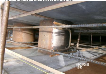
AID MCPH2 - Sta 718+00 Intake Structure head wall, (2) x 12-IN wall pipe, #4 @ 12 Vert + #4 @ 12 Horiz, TOW elev 3903.5 03-25-25
