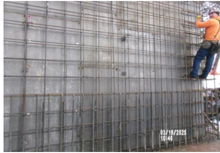
AID MCPH2 - Sta 718+00 Intake Structure outside wall reinforcing steel, #5 @ 12 Vert + #5 @ 12 Horiz (1) 03-18-25
