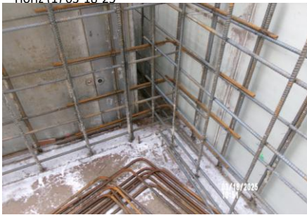
AID MCPH2 - Sta 718+00 Intake Structure t-intersect reinforcing steel, #5 @ 18 corner bar 03-18-25
