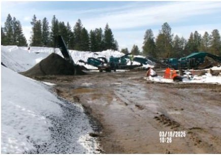
AID MCPH2 - Sta. 720+00 Temp Mtrl Processing Area, 0.75 aggregate processing 03-18-25
