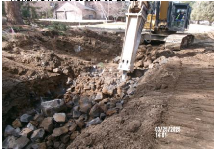
AID MCPH2 - Sta 777+20 54-IN ID profile wall HDPE pipe trench excavation 03-25-25
