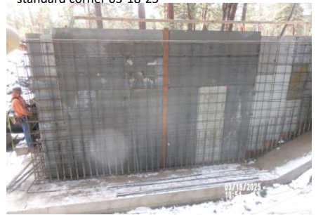
AID MCPH2 - Sta 718+00 Intake Structure outside wall reinforcing steel, #5 @ 12 Vert + #5 @ 12 Horiz (2) 03-18-25
