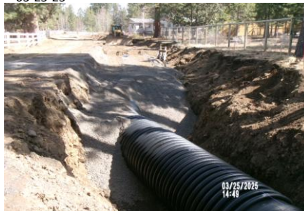
AID MCPH2 - Sta 798+75 54-IN ID profile wall HDPE pipe, initial backfill 03-25-25
