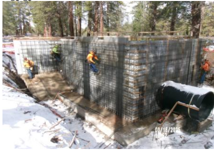
AID MCPH2 - Sta 718+00 Intake Structure head wall reinforcing steel installation 03-18-25
