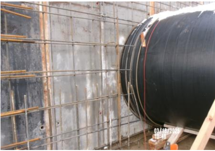
AID MCPH2 - Sta 718+00 Intake Structure head wall reinforcing steel, #4 @ 12 Vert + #4 @ 12 Horiz + (3) #4 vert @ 10 jamb and header + (2)
