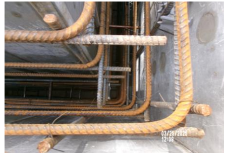
AID MCPH2 - Sta 718+00 Intake Structure form and bar, corner, #5 @ 12 corner bar, standard corner 03-25-25
