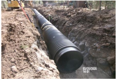
AID MCPH2 - Sta 777+50 54-IN ID profile wall HDPE pipe installation 03-25-25
