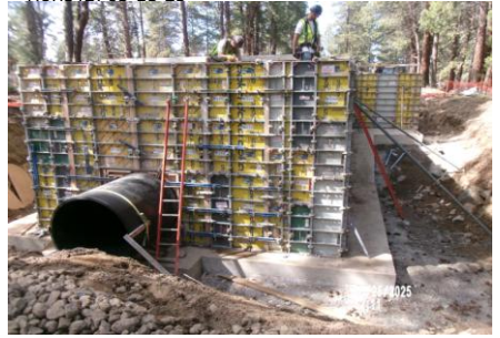
AID MCPH2 - Sta 718+00 Intake Structure wall form and bar near complete 03-25-25
